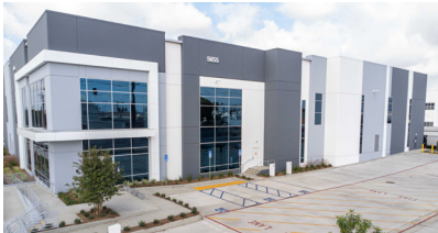
Palisade Santa Fe Center Vernon, CA Industrial
